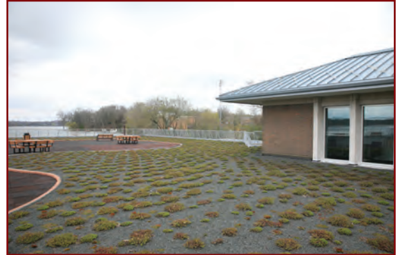
Day1: Conventional / Built in Place systems may look like this and be prone to weed infestation.
