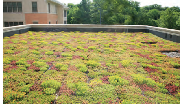
Other modular system project in June (above) & April (below)
