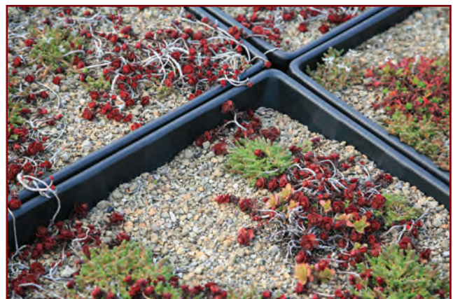
Other modular systems may have exposed lips, making them vulnerable to photodegradation and allowing for warm or cool air to escape from the building below.
