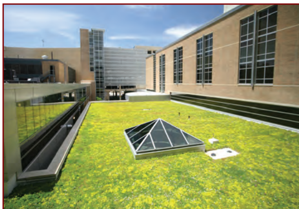
LiveRoof ® modules eliminate air gaps and are protected from harmful UV rays to prevent photodegradation.
